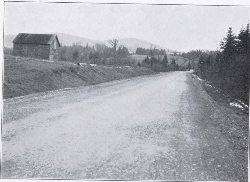
AFTER CONSTRUCTION MARSHFIELD-CABOT 27-L 7.2 Miles Macadam Surface—1932
