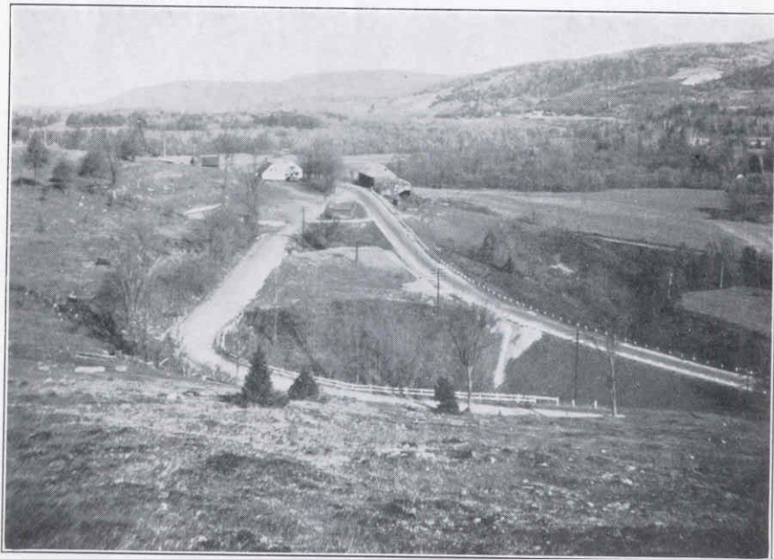
AFTER CONSTRUCTION RANDOLPH-BETHEL F. A. P. 67-B 6.1 Miles Bituminous Treated Gravel—1932
