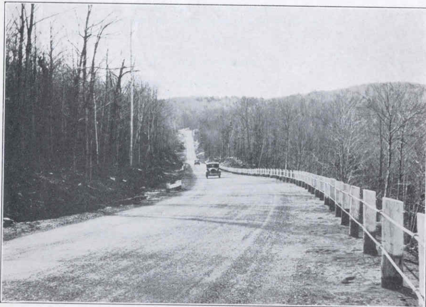
AFTER CONSTRUCTION MARLBORO F. A. P. 63-B 2.8 Miles Bituminous Treated Gravel—1932
