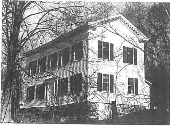
Among the several impressive Federal style buildings in West Haven is one (29) built in 1798 for Dr. Simeon Smith and believed to have been used by him as a guesthouse and dance hall. The eavesline is marked by an exceptional entablature, complete with dentils and small modillion blocks.
